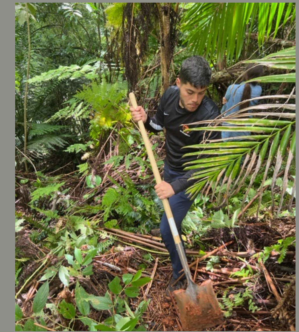
Trail restoration for flood evacuation
